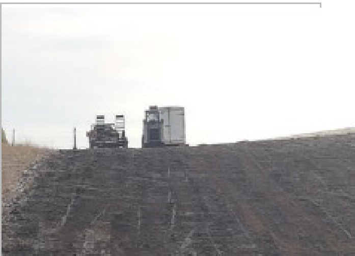
Fencing crew prepping to install fence – SF 59 – Nov 21, 2018
