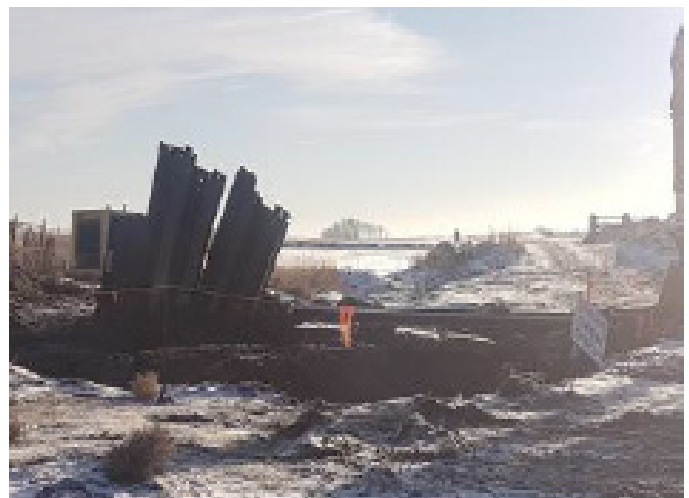
Open bellhole for valve – SF 61 – Nov 20, 2018
