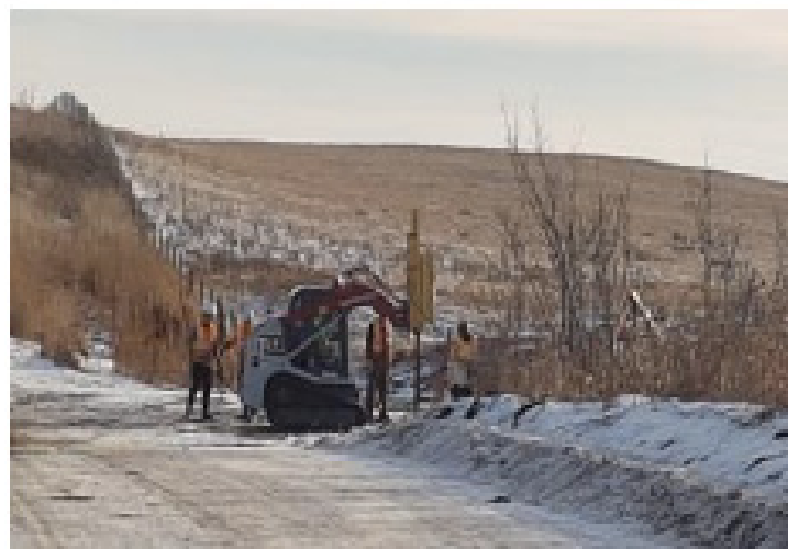
Fencing crew pounding in fence posts - SF 30 – Nov 20, 2018
