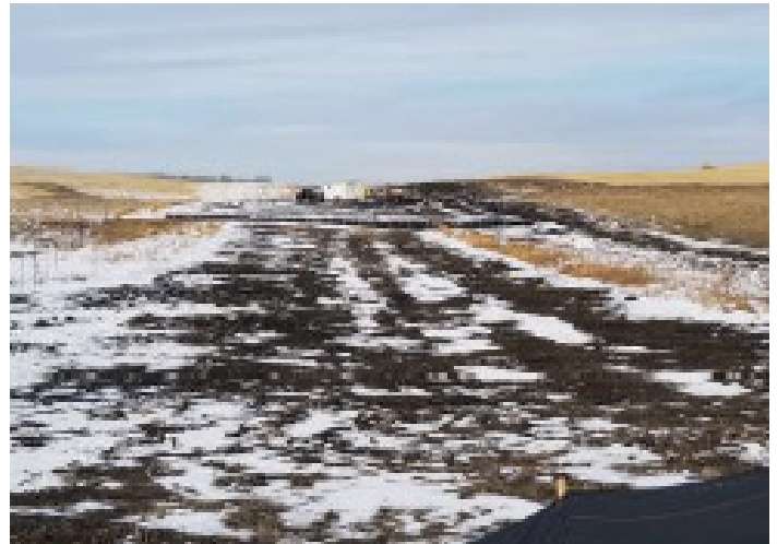
Inspect silt fence – SF 22 – Nov 22, 2018
