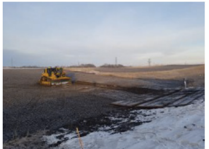
Dozers left for transport, soils are replaced – SF 35 – Nov 21, 2018
