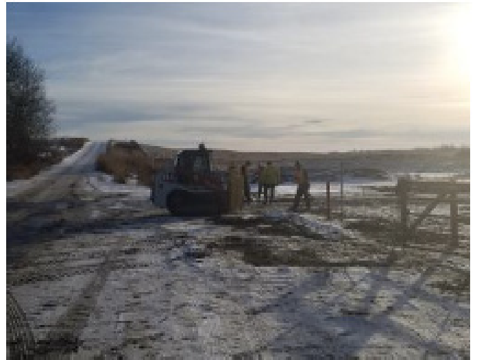
Fencing crew installing fence – SF 31 – Nov 20, 2018
