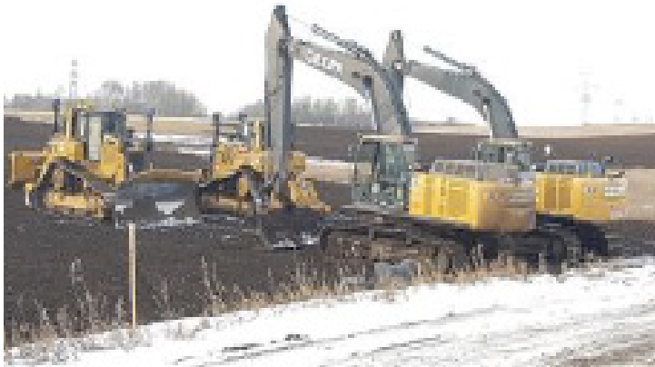
Geotec, dozers and excavators at access – SF 34 – Nov 19, 2018
