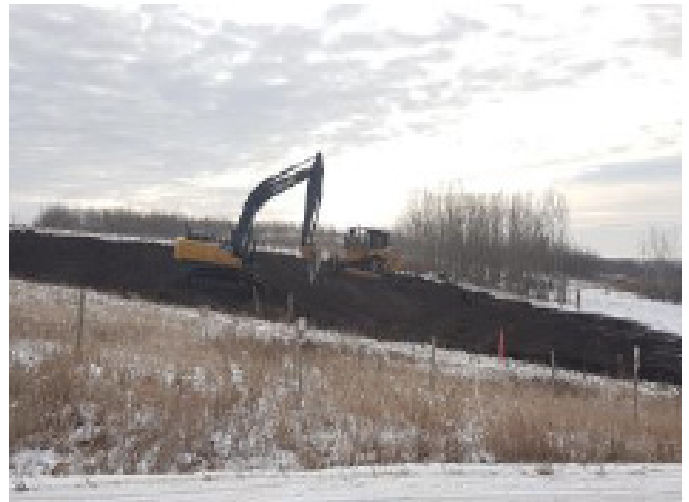
Replacing topsoil from ovality dig– SF 30 – Nov 19, 2018
