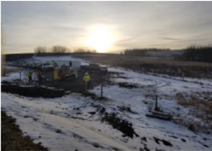
Fencing crew fixing deficiencies – SF 30 – Nov 21, 2018
