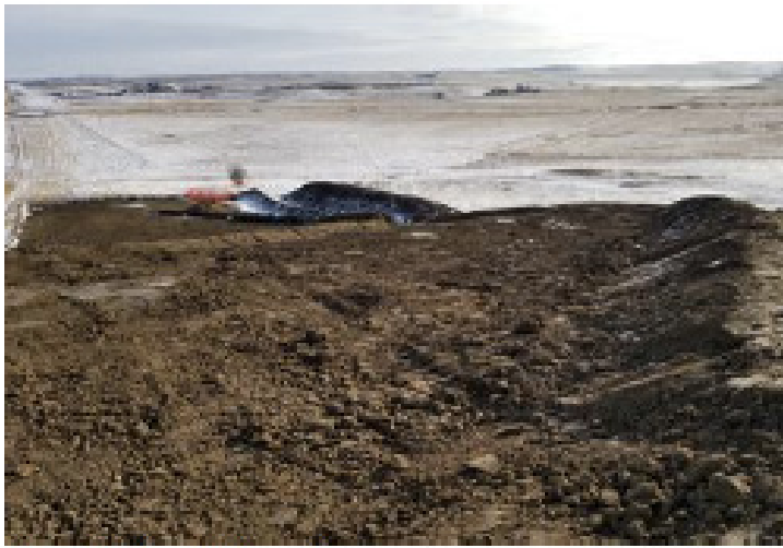
Diversion berms – SF 27 – Nov 19, 2018
