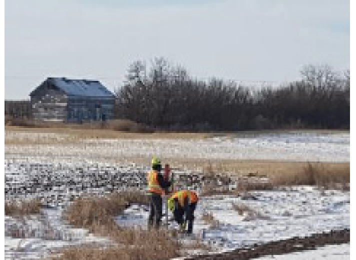
Utility crew putting in pipeline warning signs – SF 79 – Nov 22, 2018
