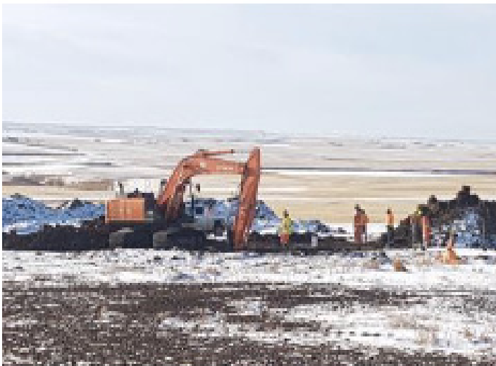
Excavator digging bellhole - SF 71 – Nov 22, 2018
