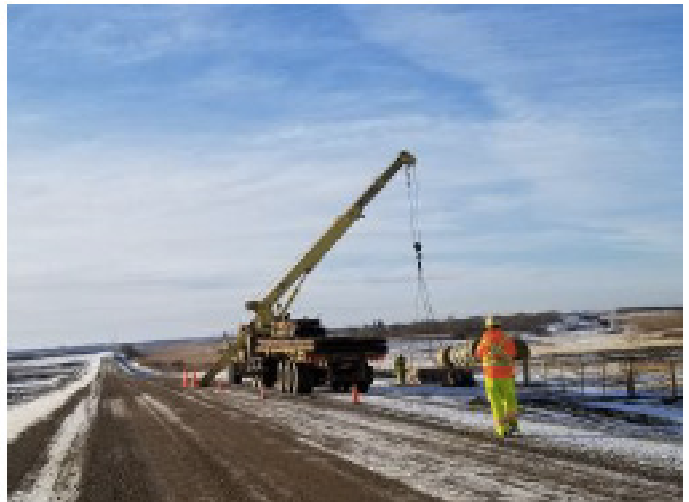
Crane removing rig matting from ditch – SF 19 - Nov 19, 2018
