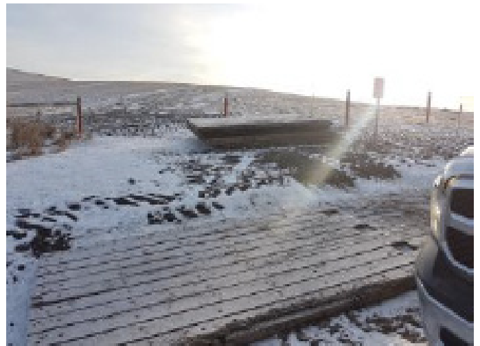
Rig mats at access road ready for removal – SF 61 – Nov 21, 2018
