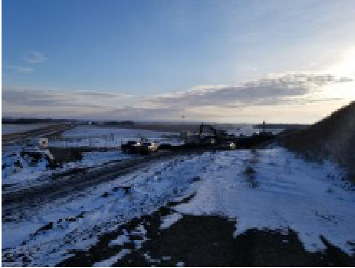
Excavator shading pipe, crew working on valve site– SF 59 – Nov 23, 2018
